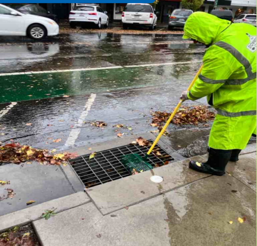
Ambassadors in Action Clearing Storm Drain
